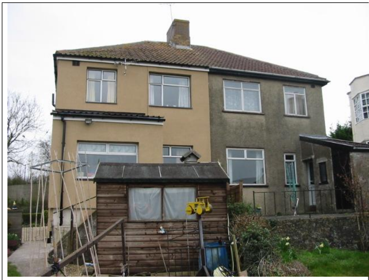
Figure 13. SWI improves the appearance of the home as demonstrated by C20's completed installation in comparison with the other half of the semi-detached dwelling.
