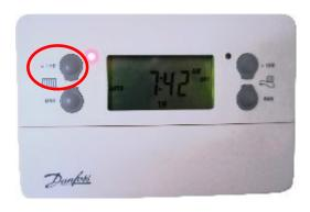
**Boost** or **+1hr** puts the heating on for an extra one hour of heat.
