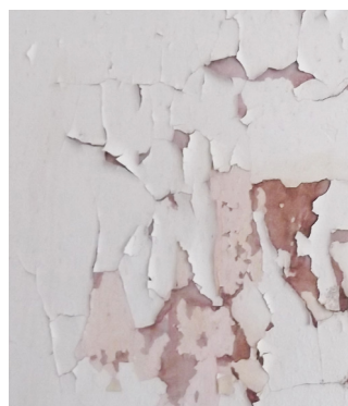
Left: Penetrating damp can cause paint to flake. Right: Rising damp in wall can look like this, but can be difficult to diagnose.
