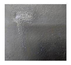
When moist air reaches cool surfaces like walls it turns back into water and makes them damp.
