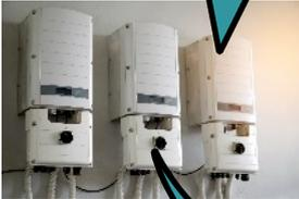
The **inverter** takes electricity from the panels and changes it so it can be used in the home.
