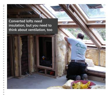
insulation is consistent throughout the loft, so that there are no cold spots (or 'thermal bridges').
