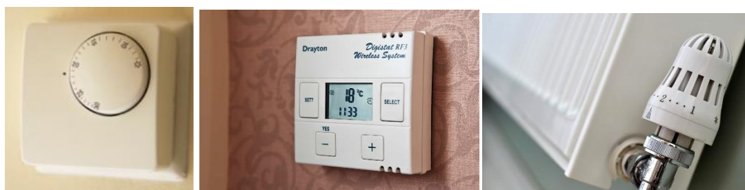
Thermostat (left), timer/programmer with thermostat (middle), TRV (right)
