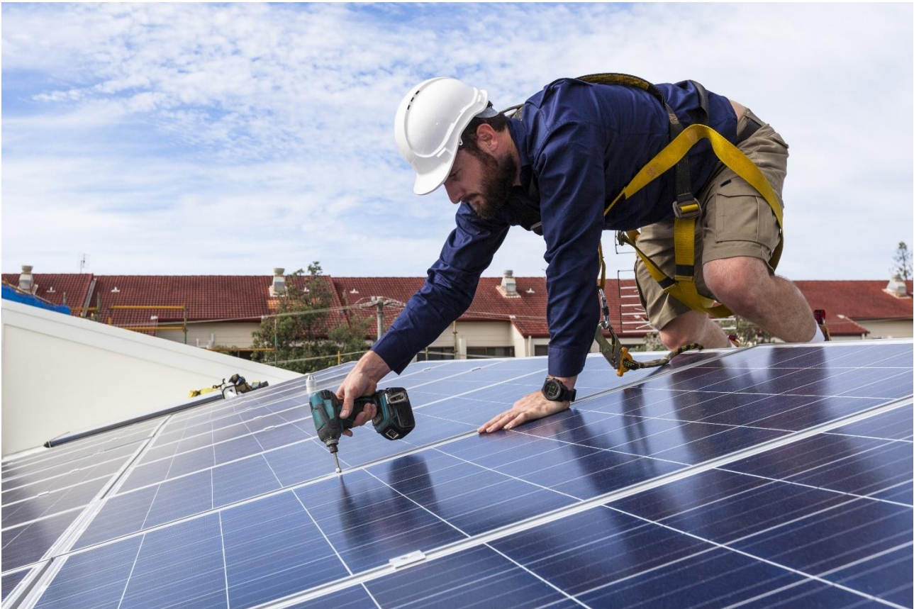
Fitting a solar PV array to the roof of a home.
