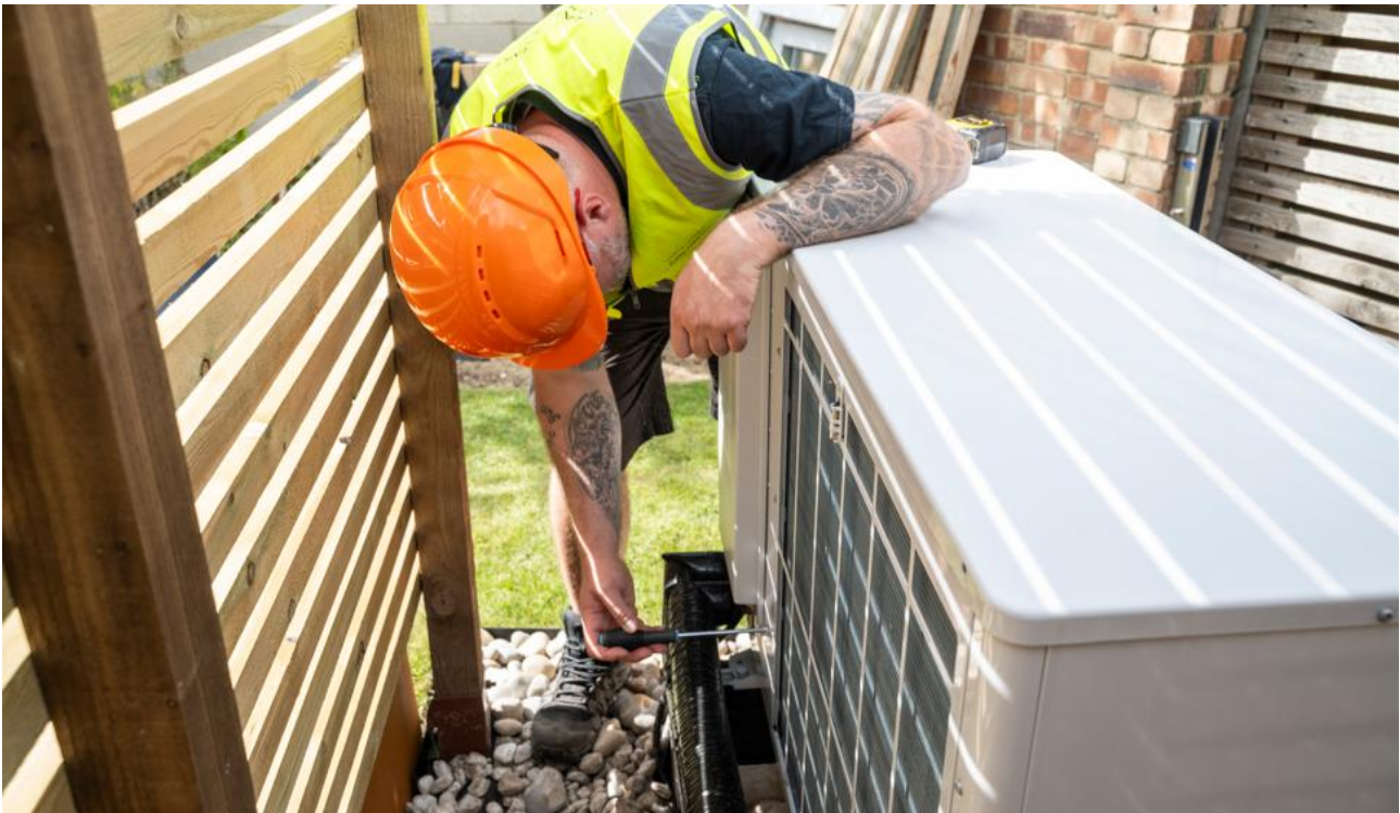
An installer fits a heat pump.
